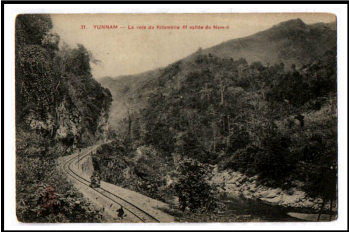
Section of rail line at kilometer 41.
