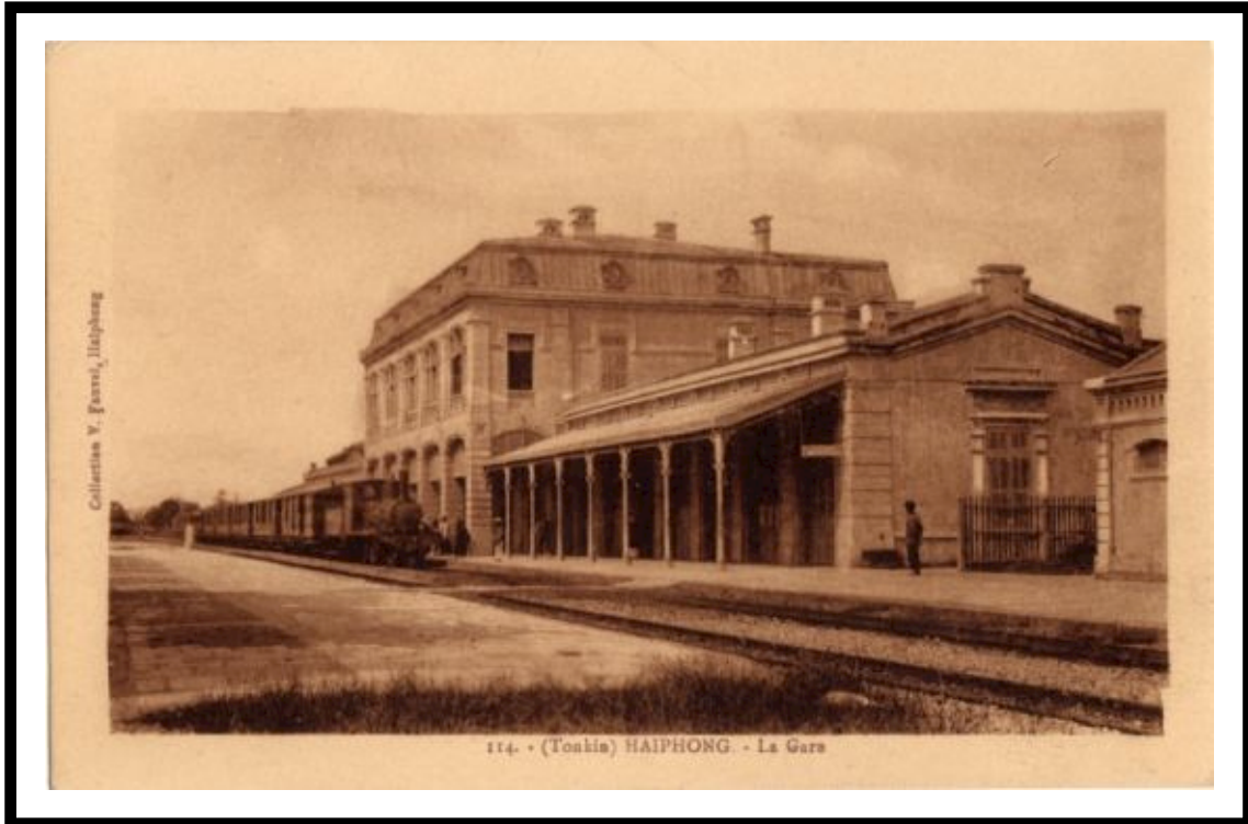
Haiphong Train Station
