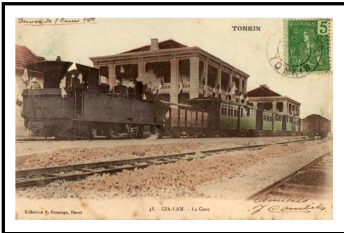
Gia-Lam Train Station
