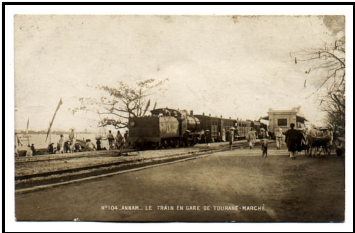
Tourane Train Station
