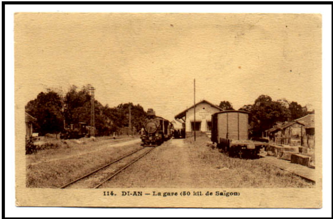
Di-An Train Station
