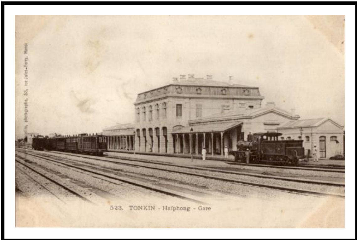
Haiphong Train Station
