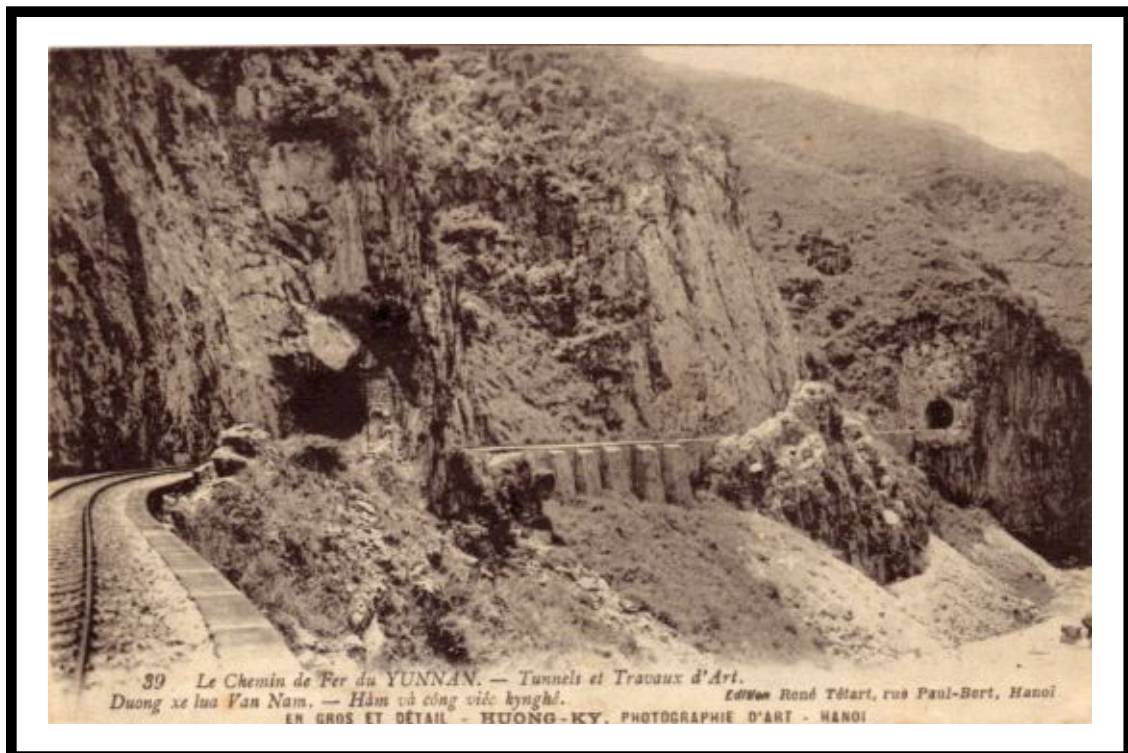
The rail bed had to be reinforced to support the enormous weight of trains.
